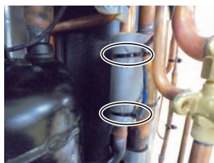
Thermistor (Discharge)
